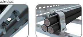
5. Place the cable into the cleat option and pull the hinged arm over the cables.
